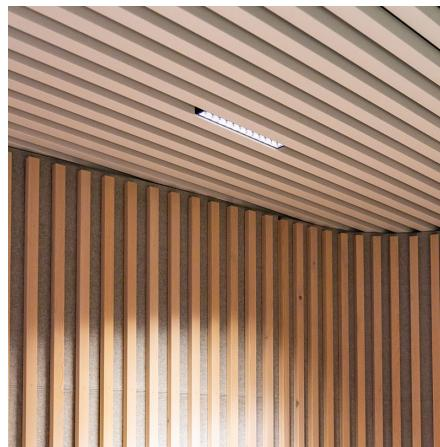
Evolo-L is an elegant, slim LED fixture featuring a row of mid-power LEDs, each with its own lens and louvre. This fixture is specifically designed for use in linear panel ceilings.
