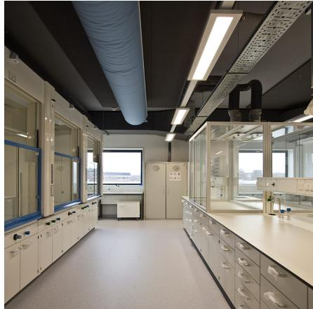
Fusion-C is a surface-mounted luminaire suitable for both general lighting and effective task lighting. The LED luminaire was developed as an alternative to T8 and T5 linear fluorescent luminaires for use in both renovation and new construction projects. The luminaires are made of a slim metal housing finished with a matte white powder coating.
